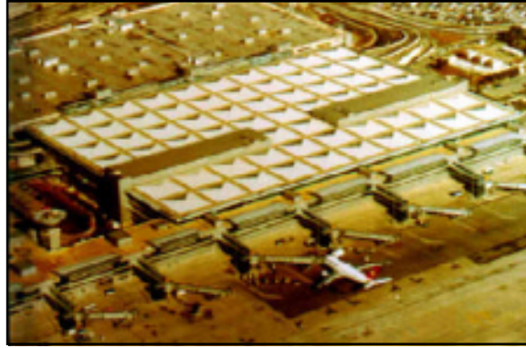
■ Figure 1. New Ataturk International Airport Terminal Building
