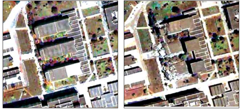
Before (left) and After (right) pan-sharpened Quickbird images of the Bourmedes, Algeria earthquake of May 2003 showing building damage.
