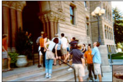
■ Dr. T. Leslie Youd led a field trip to several seismically designed or retrofitted buildings in the Salt Lake City area. Shown above is the historic city and county building, which was retrofitted with base isolators.
