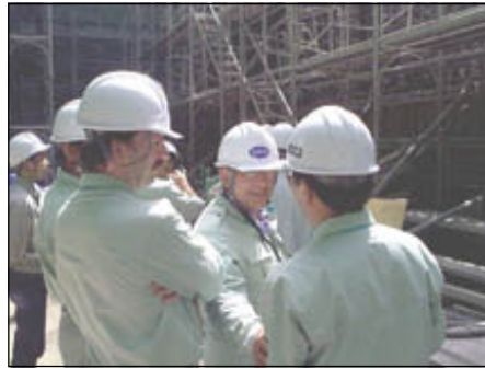
■ Profs. Bruneau and Reinhorn discuss progress with engineers at the construction site of the National Institute for Earth Science and Disaster Prevention (NIED) Jumbo Shaking Table at Miki City, outside Kobe.
