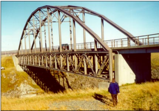
■ The Thjorsa bridge in the South Iceland Lowlands was subjected to a peak ground acceleration of 0.84 g.
