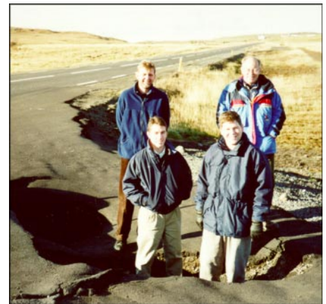
■ The investigative team is pictured standing inside a large surface crack in a parking lot in Skeidar. Front row: M. Higgins and B. Bessason; back row: G.I. Balduinsson and E. Hafliðason.
