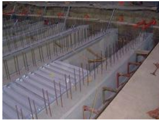
Figure 2.3.3. Photo of Stay-in-Place Metal Deck Form
