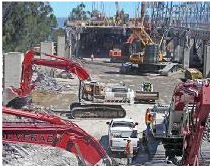
Figure 3.1.1. Photo of Bridge Demolition
