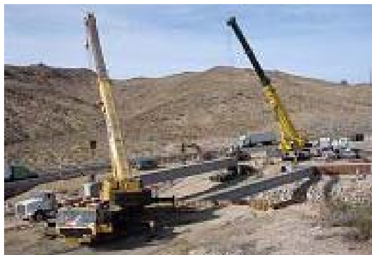
Figure 2.1.4. Photos of Precast Girders Placement
