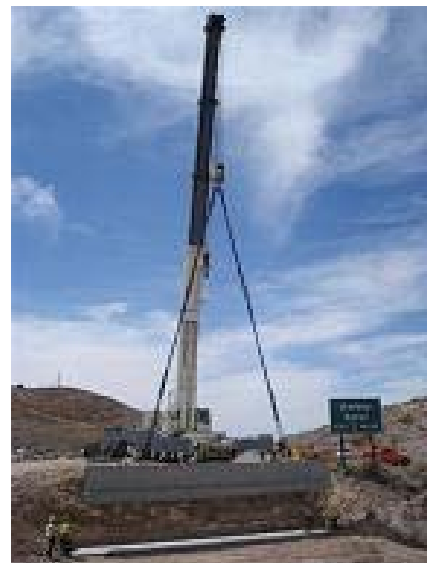
Figure 2.1.2. Photos of Precast Abutment Placement
