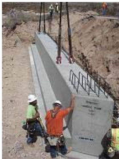
Figure 2.1.2. Photos of Precast Abutment Placement
