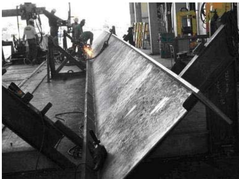
Figure 2.2.7. Girder Fabrication at Stinger Welding
