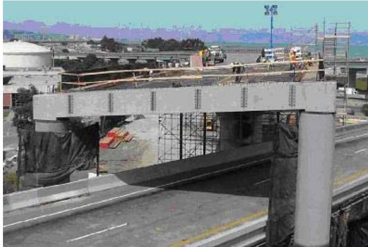
Figure 2.2.8. Completed Concrete Bent Cap
