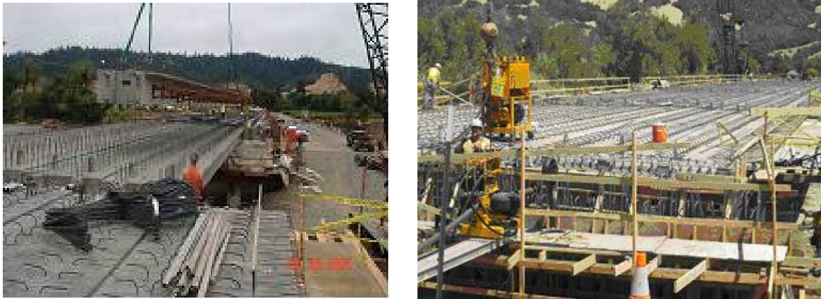
Figure 2.4.5. (b) Construction Photos
