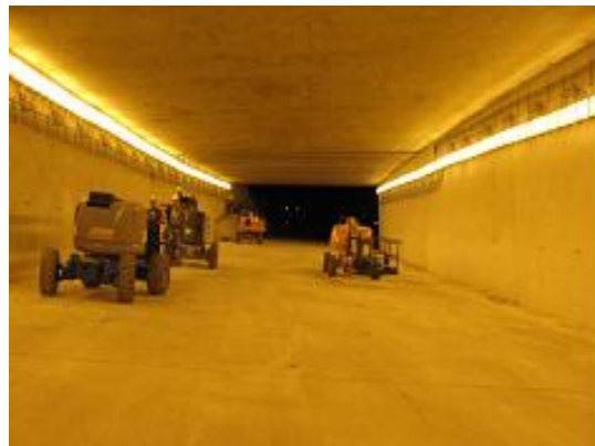
Figure 2.3.4. Photo of Construction Completion
