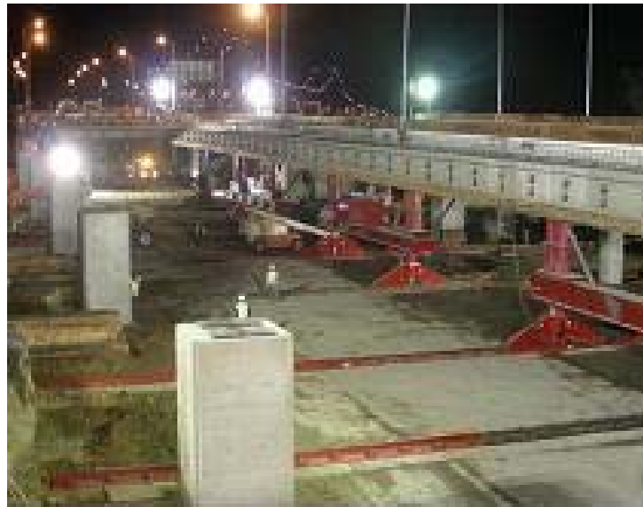
Figure 3.1.2. Photo of New Bridge Roll-in
