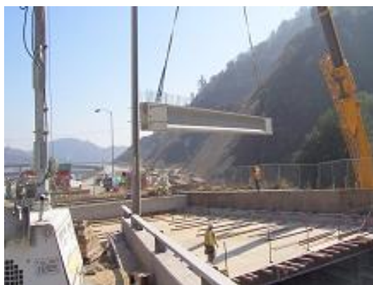
Figure 2.3.2. Photo of Girder Placement
