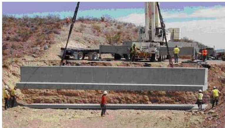
Figure 2.1.3. Photos of Precast Abutment Placement
