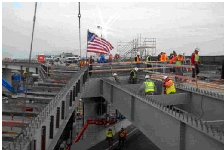
Figure 2.2.9. Last girder installed at the jobsite
