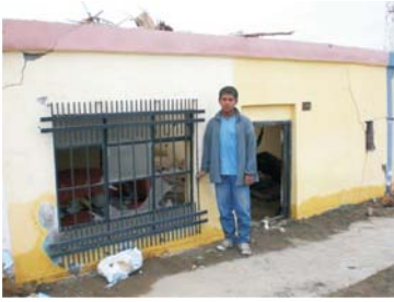
Settlement of some 2.6 feet (0.8 m)
